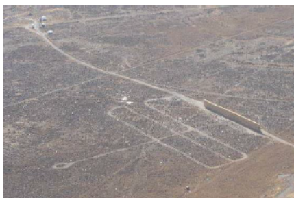
Figure 2: Aerial view of the mock sound barrier (6m height, 90m length) test site. Source: /CLA09/
