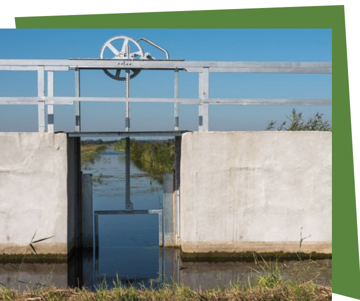
Rehabilitated weir in a ditch for rewetting a fen
