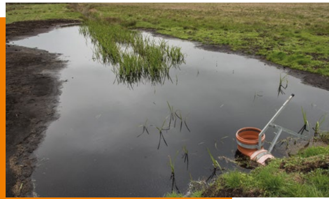
Rewetting measure by installing an adjustable ditch gate
